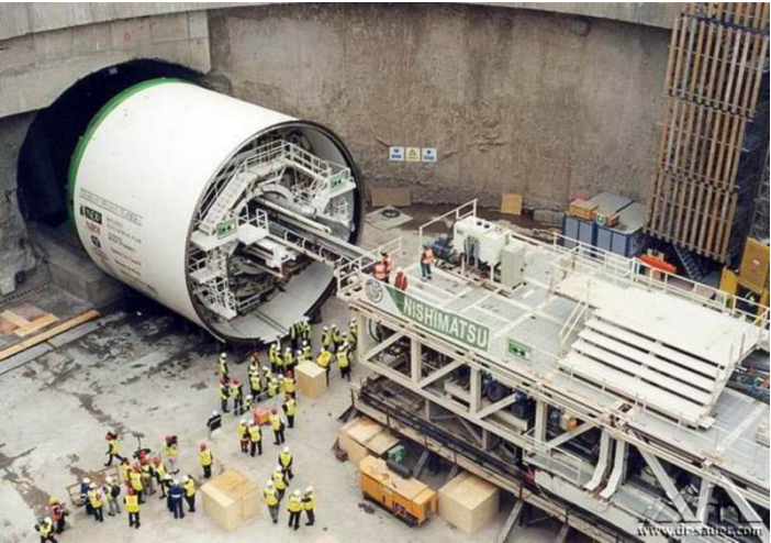
TBM - Dublin Port Tunnel
